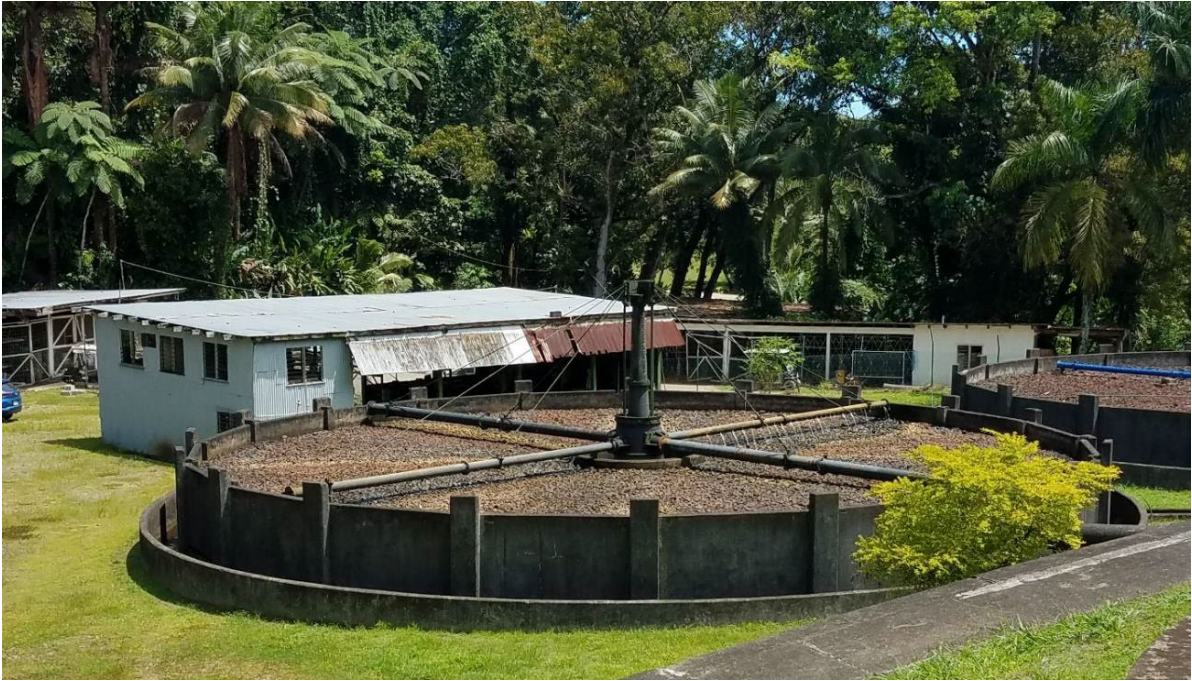
Figure 3: Trickling Filter and office building at Pacific Harbour WWTP
